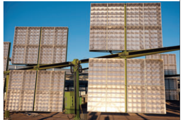
CPV SYSTEMS with dual-axis trackers are one of five solar technologies in use at Arizona Western College.
