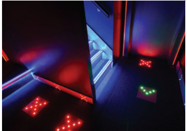
AT UPPER IOWA University, a new "intelligent" emergency lighting system guides evacuees to the nearest escape route.
